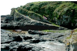
Slipway at Bessy's Cove
