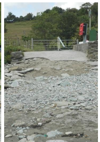
The slipway to Talland Sand
