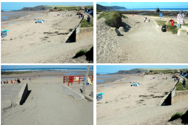
The slipways and various views of the Black rock area of the beach
