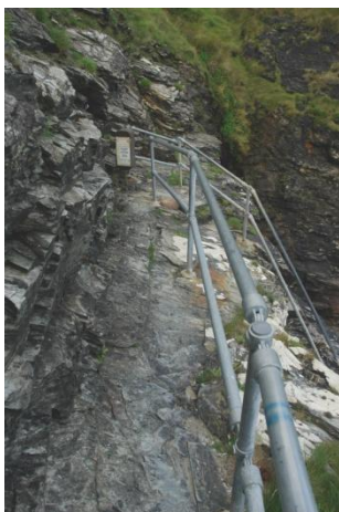
Access path down the cliffs
