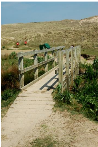
Bridge across the stream
